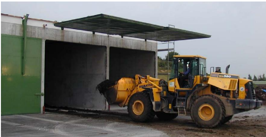
Picture 1: Garage-type Fermenter (Pietzsch, 2007)
