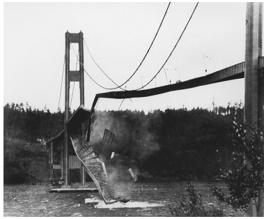
(a) Tacoma Narrows Bridge Collapse (Encyclopaedia Britannica, 1940)
