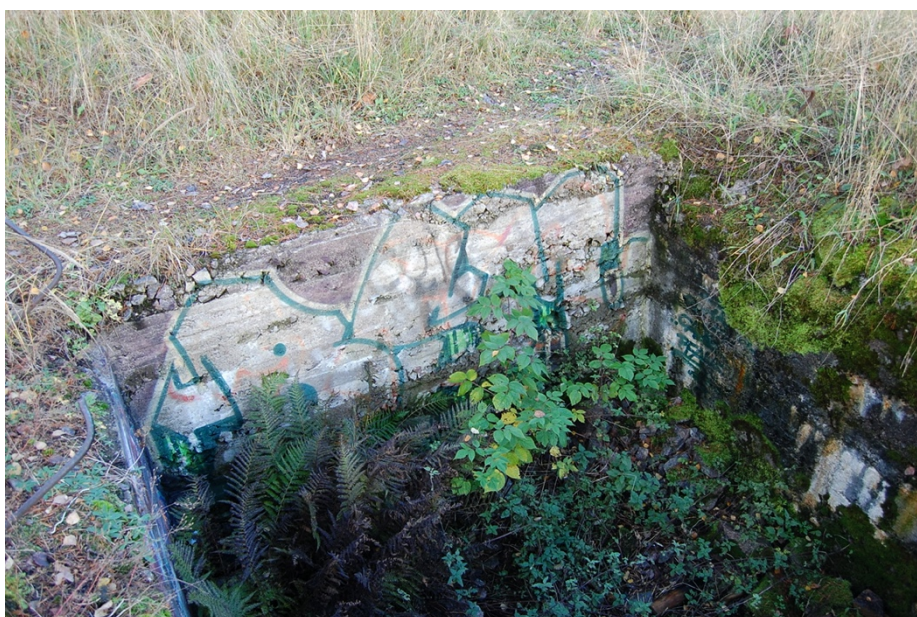
FIGURE 31 Spray-painted dugout walls at Vartiokylä Hill Fort in 2012. Photo: Heidi Wirilander 2012.
