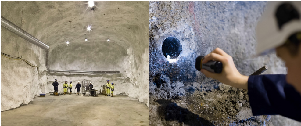
Figure 4. Left: the experimental hall of Callio Lab2 after its completion in the spring of 2016. The area is about 120 m 2 . The maximum height is 9 m. Right: example of a borehole originating from Callio Lab2. The diameter is 7.5 cm. Typical length is about 700 m. Due to the high quality of the rock, the inner surface of the hole is smooth, facilitating deployment of instrumentation. The photo was taken before the walls of the main hall were painted.
