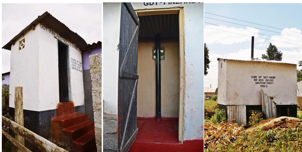
Picture 3. Several urine-diverting dry toilets have been constructed in Madimba during the sanitation projects. On the right, a pile of dried fecal matter has been emptied from the toilet.
