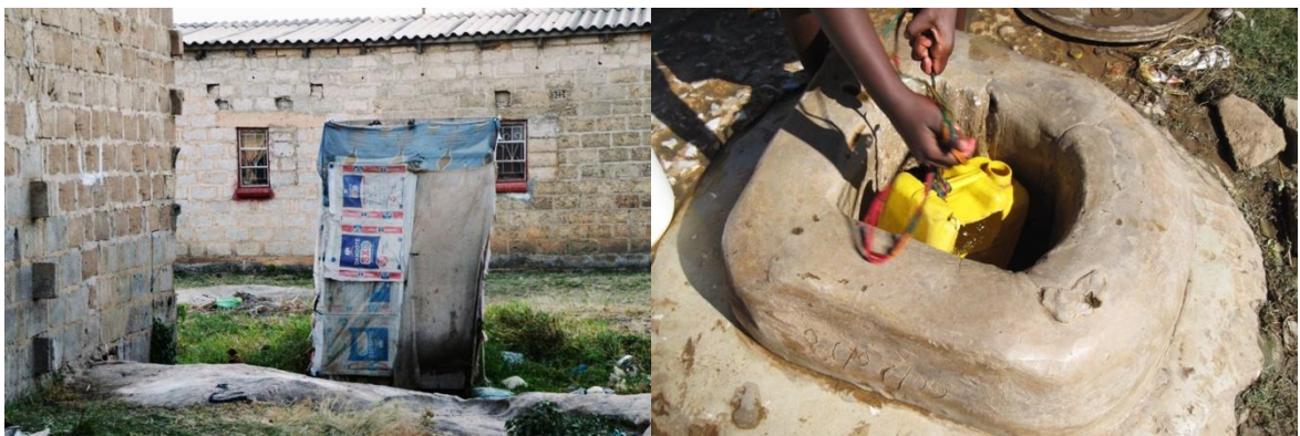
Picture 1. Pit latrines and hand-dug groundwater wells are common water supply and sanitation facilities in Zambia.
