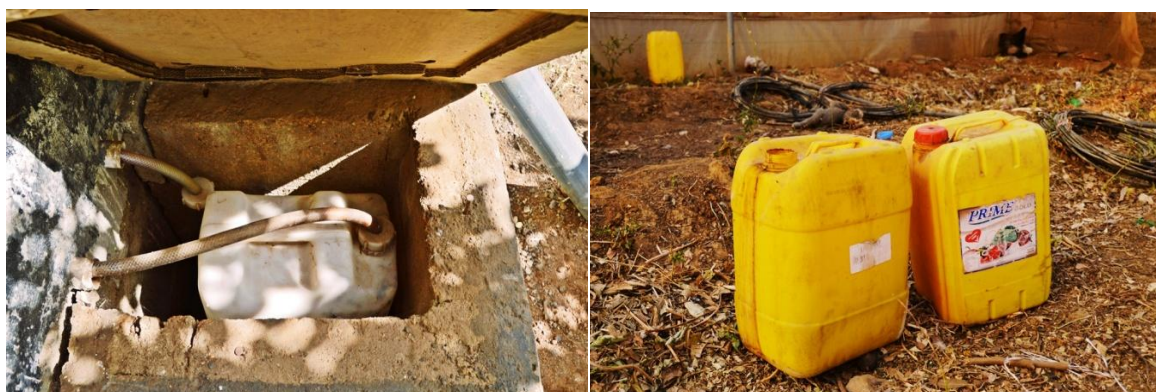
Picture 4. Urine is often collected through a pipe into a plastic container stored behind the separating toilet, and stored in similar containers for at least 6 months before application.
