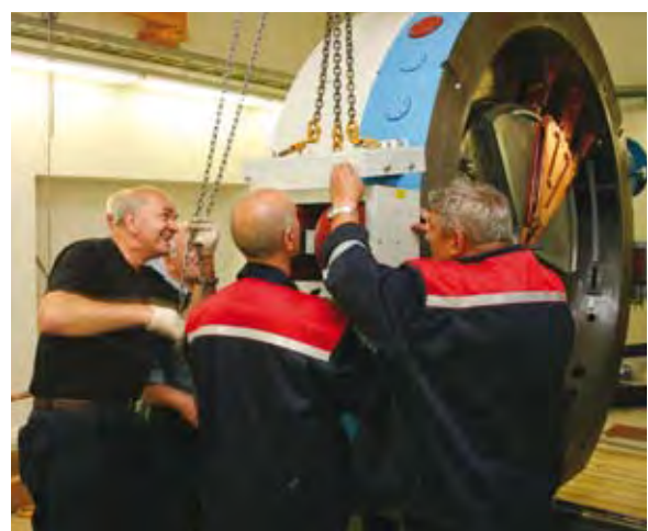
Fig. 3. The group from the Efremov Institute (NIIEFA) is installing the cyclotron components.
