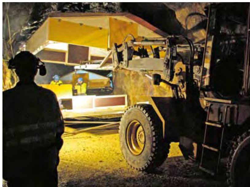
Fig. 2. Construction of underground village to house EMMA detectors
