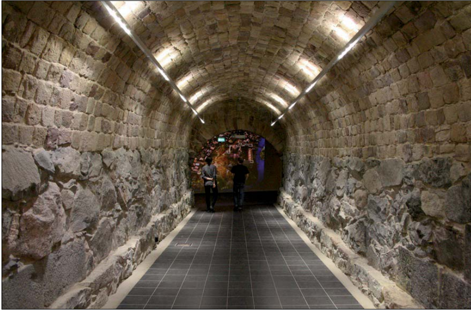
PIC 4.7 The redesigned entrance tunnel to the exhibitions of the Museum of Medieval Stockholm. The passage is lighter, both as more clearly lighted and as a bodily experience; the weight of the walls and time has been lifted.
