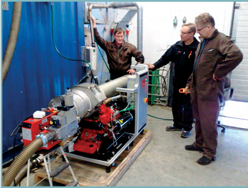
FIGURE 2. SOLO Stirling 161 micro CHP-module (9 kWe and 26 kWth) installed at the Centria renewable energy research laboratory (above) and Centria downdraft gasifier (left).
