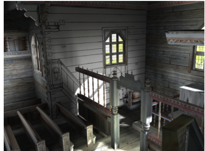
Figure 4. The drawing on the wall shows the size of the current window as compared to the original window.
