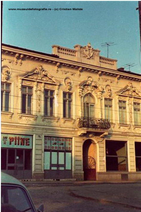
Figure 11. Museum of Photography. Cauzasi area – demolitions in 1985. Taken 27.02.2012
