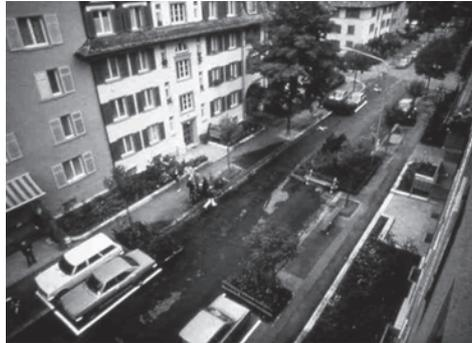
FIGURE 21 A parking layout creating chicanes to slow the vehicular traffic in Germany ('80); (La città possibile, n.d.)
