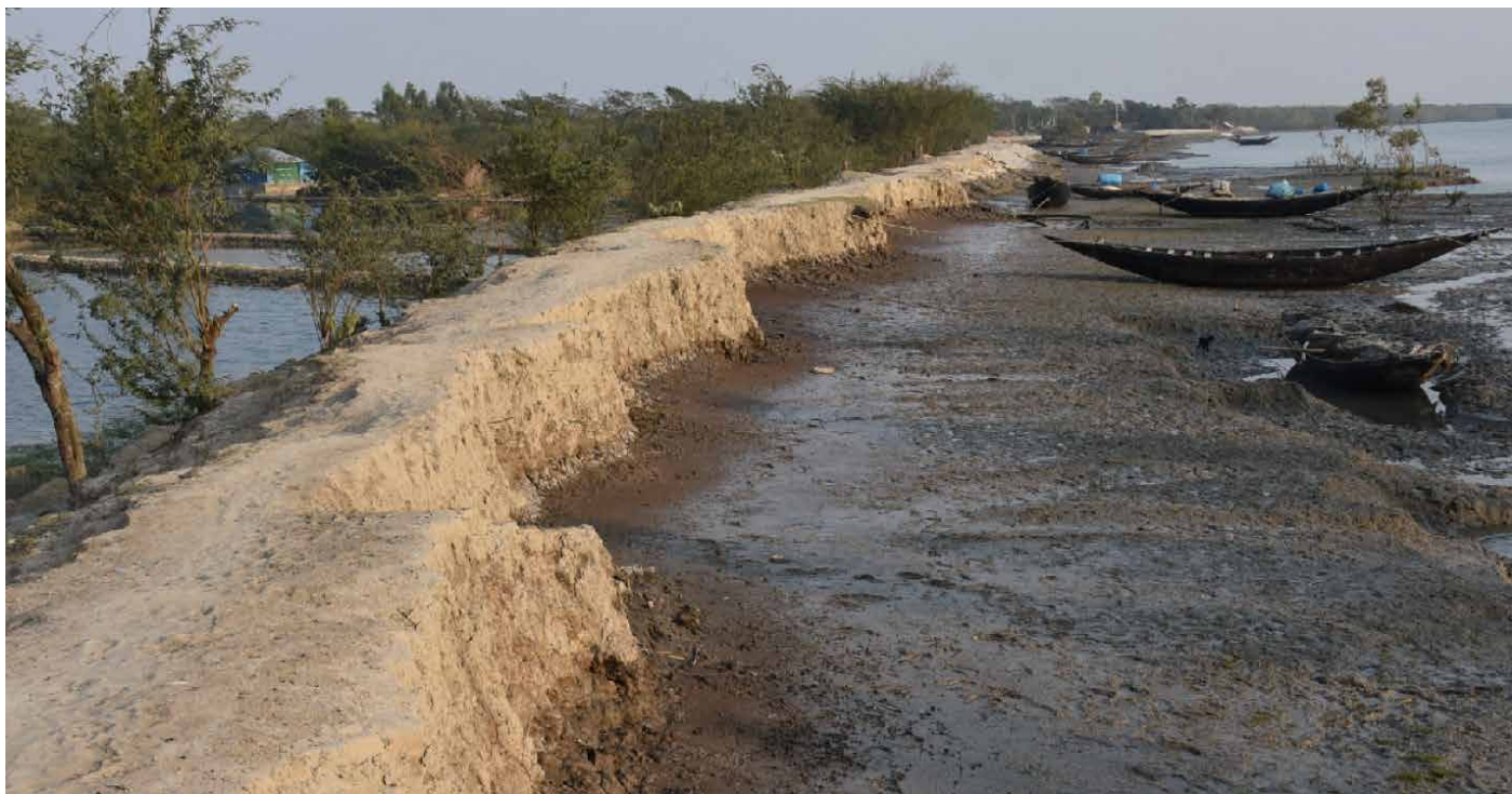
The embankment in coastal Bangladesh is not durable nor sufficient for protecting people from the surges of seawater.
