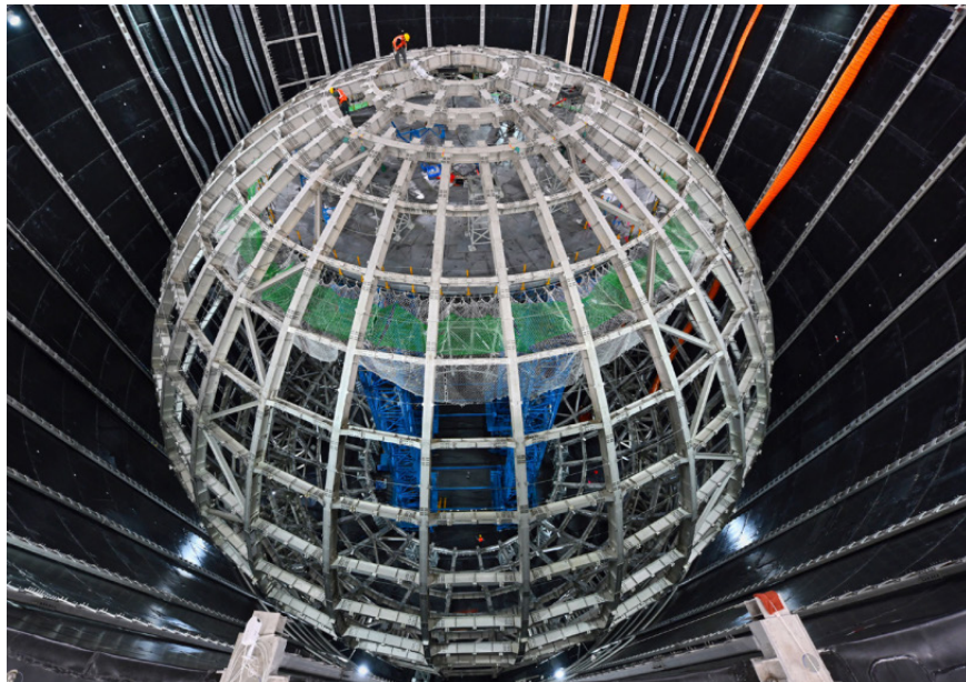
↑ Figure 1. JUNO & OSIRIS. Left: a June 2022 photo of the steel structure to support 35 m diameter acrylic globe holding 20 kton of LS. Right: OSIRIS sketch; the 3 m diameter, 3 m tall cylinder tank will sample each 20-ton batch of LS.
