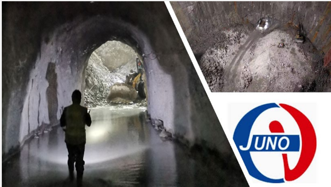
↑ Figure 2. Excavation of JUNO underground infrastructure
