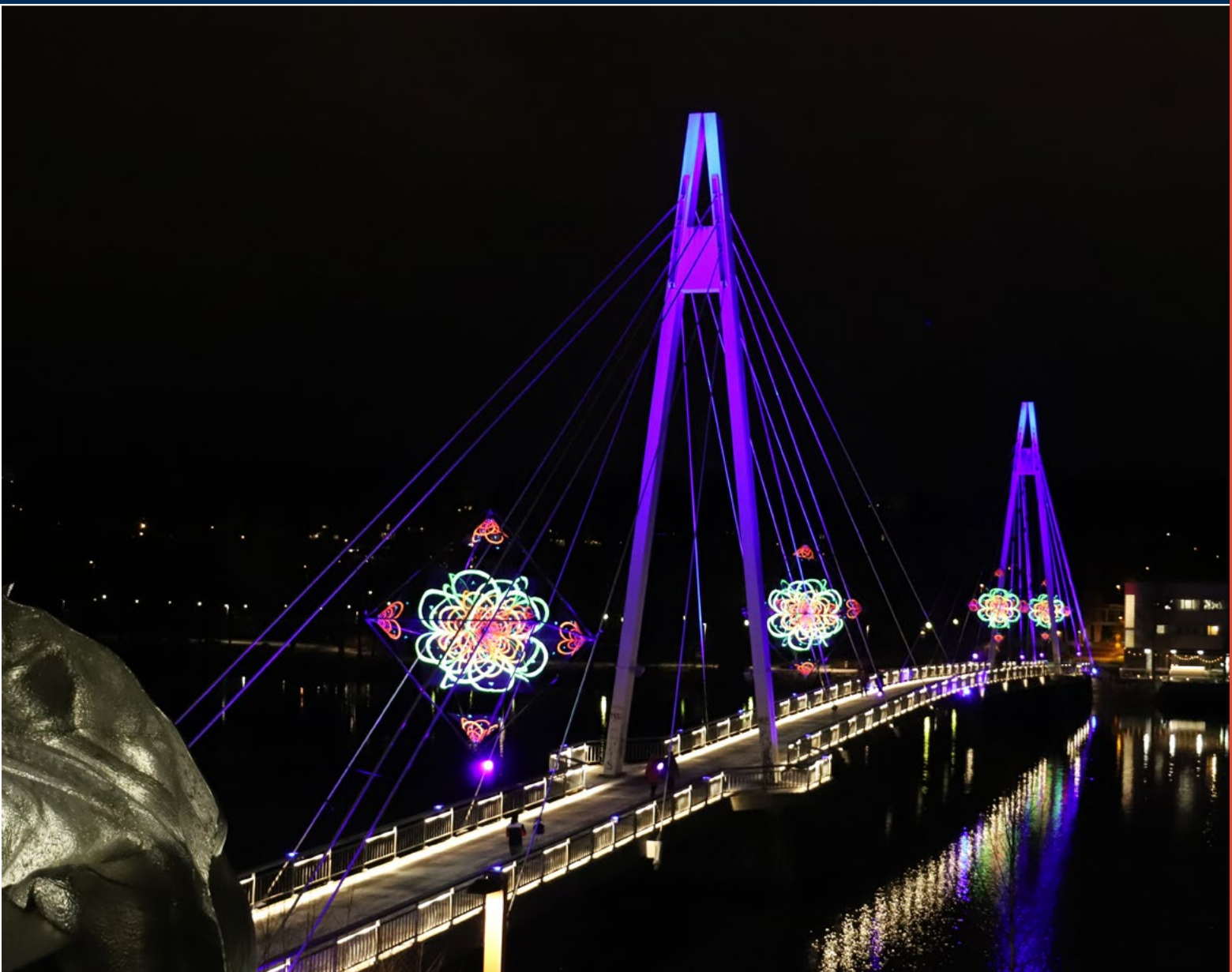
↑ Light installation at Ylistö bridge
