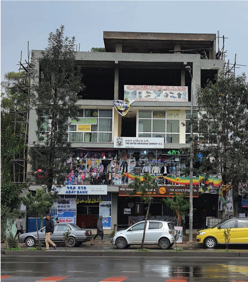
Figure 3.3 Iddir-owned mixed-use building with upper floors incrementally constructed so that one or two floors can be used for income generation ( photos by the author ).
