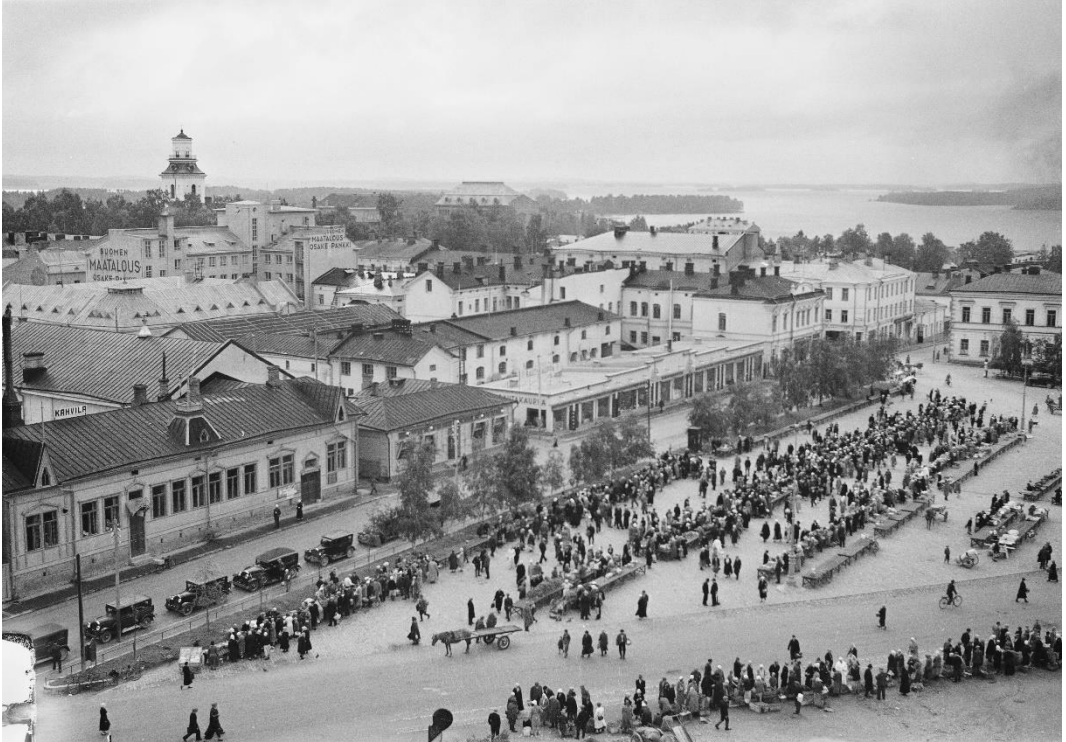
Photograph 1. Looking across the time-square.
