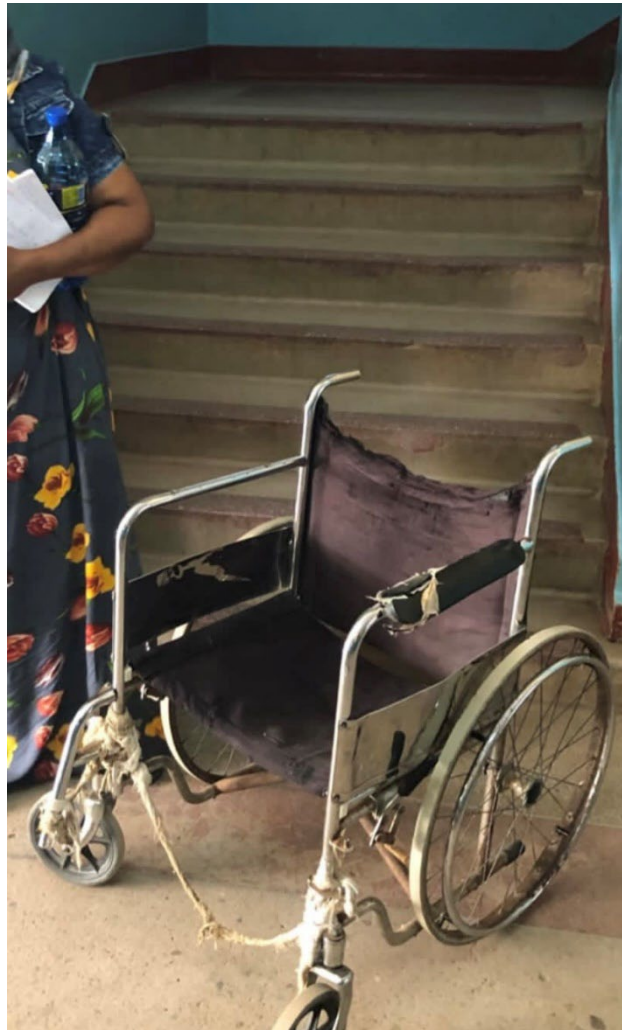
Figure 5 Inaccessibility of the second-floor maternity ward at a study site.
