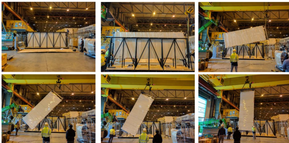
Figure 70. Arrival of an APA in EHN1 and its positioning. The upper left image shows the orientation of the APA as delivered, the lower right shows its vertical orientation when it is lowered into the material sas.
