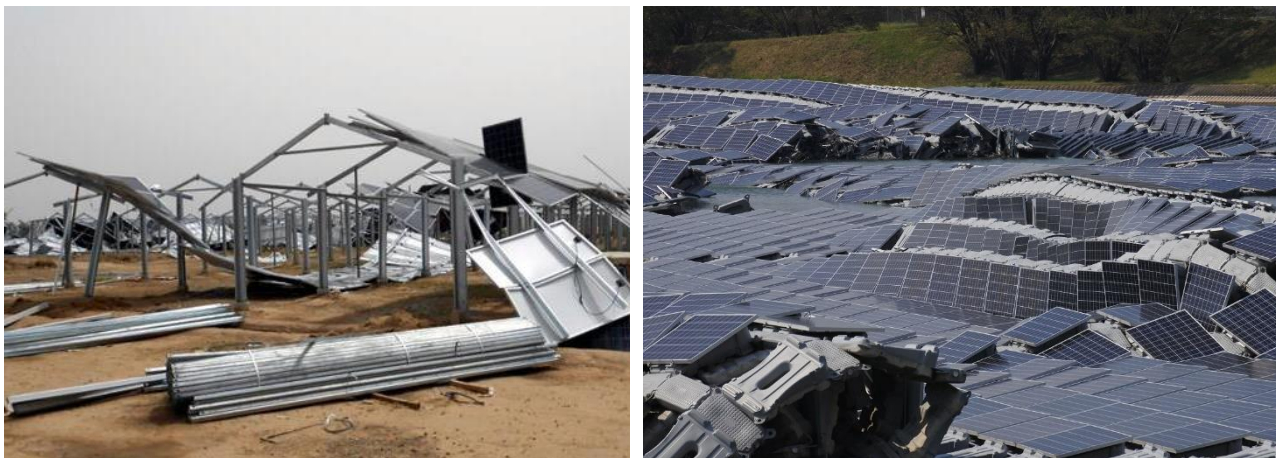
Figure 1 Effect of wind gusts on PV Modules positioned on a set of canopies (left) and an FPV plant (right)
