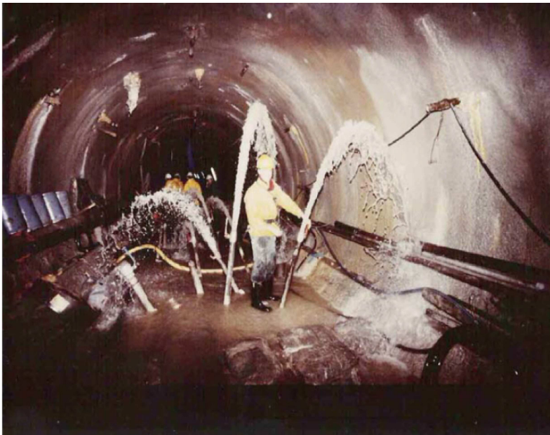
Fig. 4.10. Water inflows during LEP tunnel construction.
