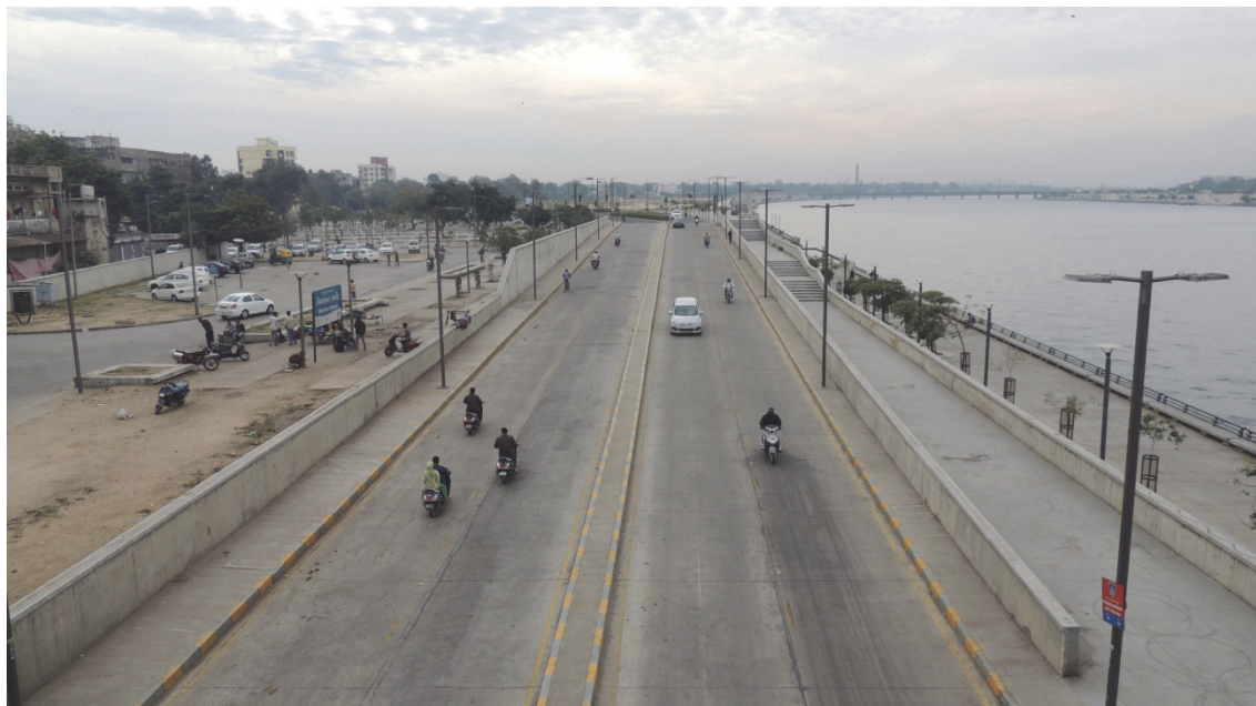
FIGURE 4.6. Rickshaws have been banned from the riverfront roads, December 2017.
