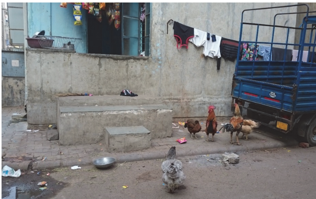
FIGURE 6.5. Concrete stairs outside a balcony that functions as a kiosk, December 2015.
