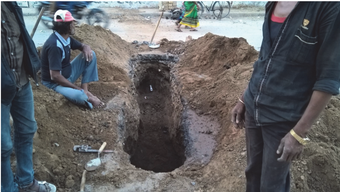
FIGURE 6.9. Building a water connection, January 2016. © Niklas Salmi
