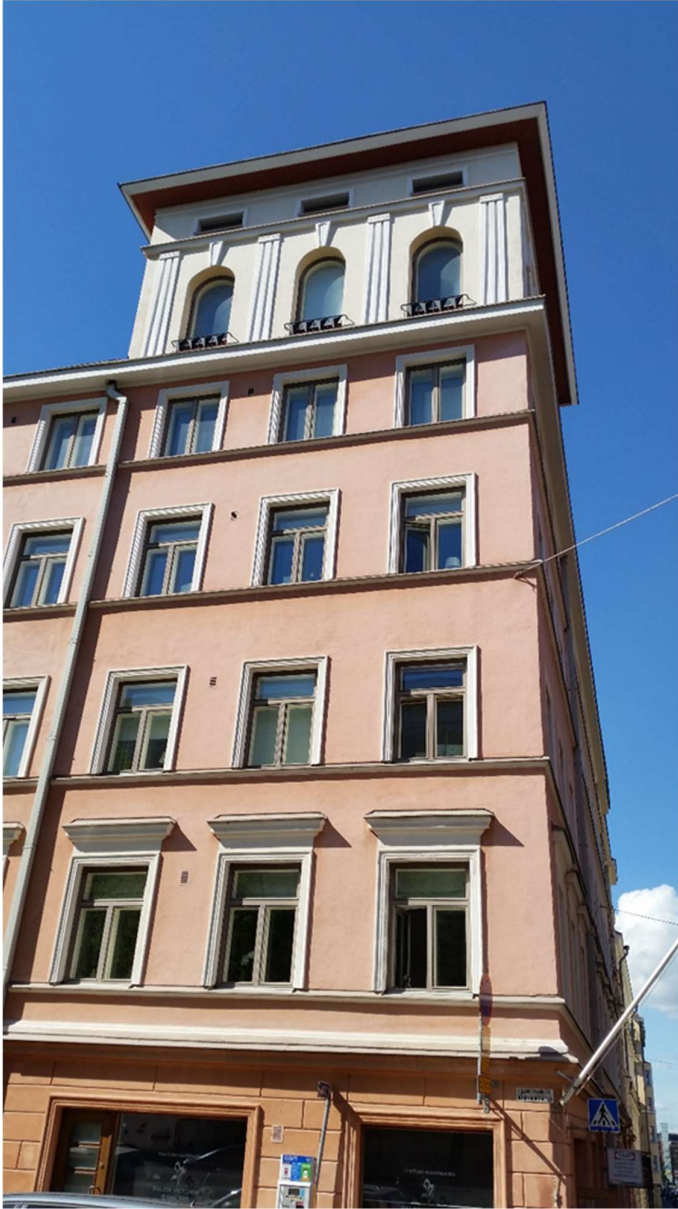
Figure 5. Apartment block where Jansson lived in her tower studio. Photo by author, 2017.
