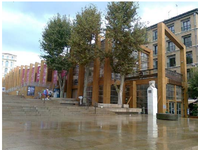
Figure 2.9. The M Pavilion, designed by Philippe Malta, in Marseille, France, in October 2013. Photo: Tuuli Lähdesmäki.
