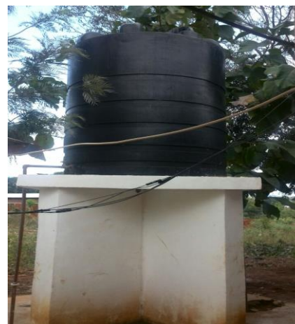
Plate 6: A water tank (5000L) connected to the water purification unit Source: MWAKANGALE (Sept. 2014)
