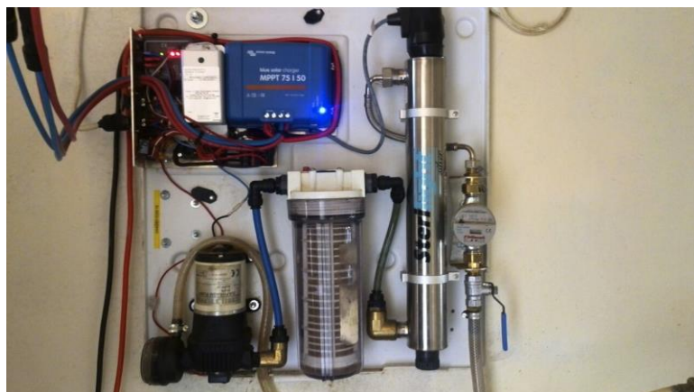
Plate 5: A composition of a water purification unit Source: SolarWAVE Company Limited, Dar es Salaam-Tanzania
