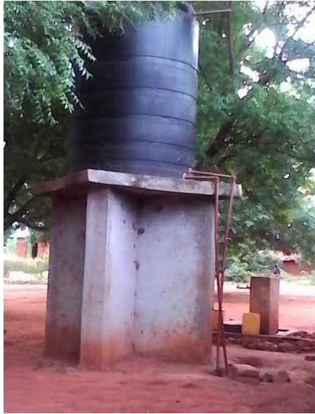
Plate 10: A water tank (5,000ml) connected to the water purification system Source: MWAKANGALE (Nov. 2014)
