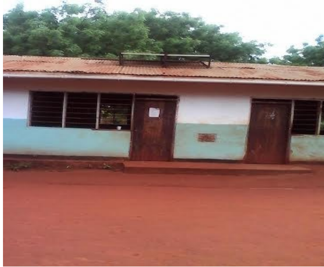
Plate 2: Vikenge Primary School Site Source: MWAKANGALE (November, 2014)
