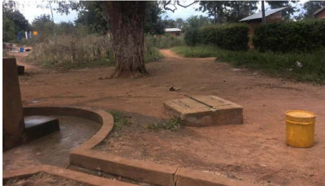
Plate 1: Community water point that does not use WP700 Source: MWAKANGALE (Sept. 2014)
