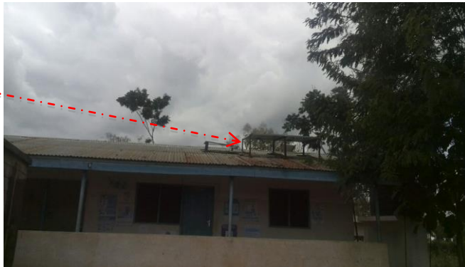
Plate 3: A solar panel installed on a roof Source: MWAKANGALE (Sept. 2014)
