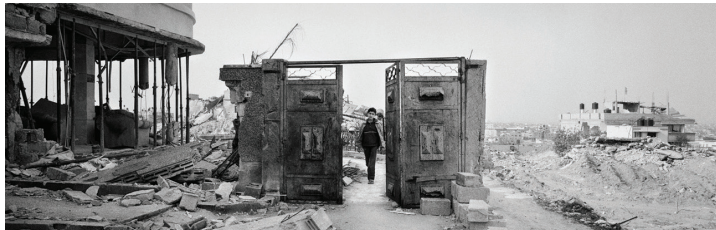
Figure 4.1. Photo Story #3 Gaza - Landscape of Destruction
