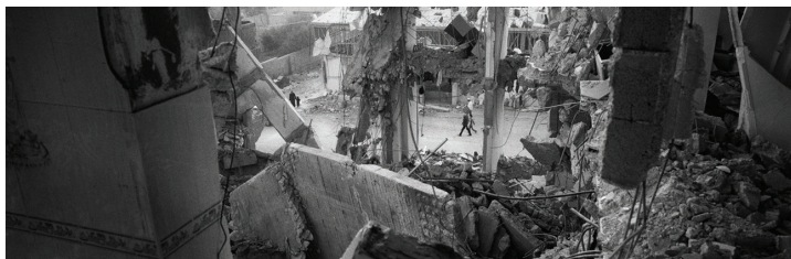
Figure 4.2. Photo Story #3 Gaza - Landscape of Destruction
