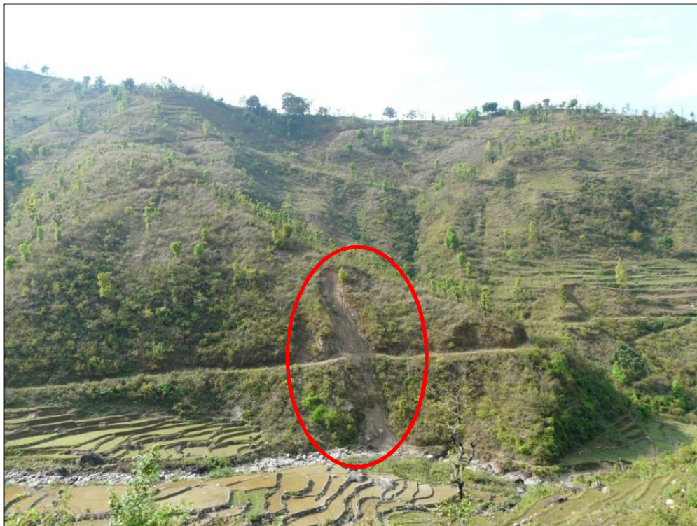
Figure 5. Road damaged by a landslide along the way to Ruchang village.
