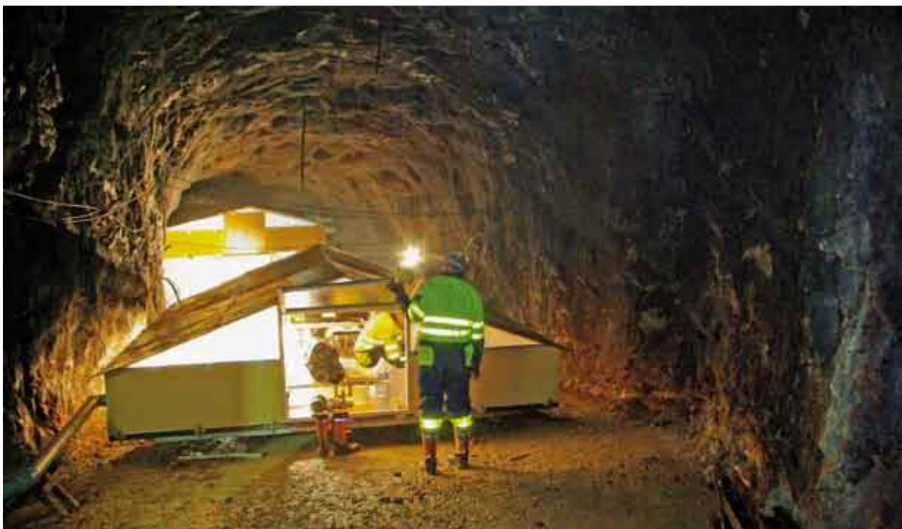
Fig. 2. Installing equipment in the underground cottages of EMMA experiment.
