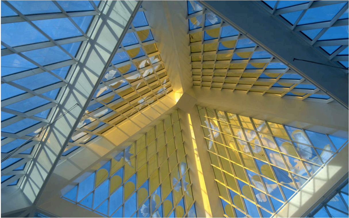
Upper Roof of the Pyramid, Foster + Partners 386
