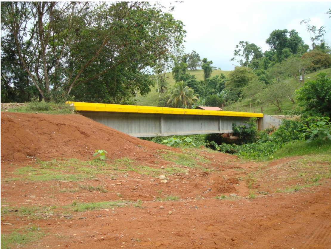
Photo of a bridge constructed by IISA
