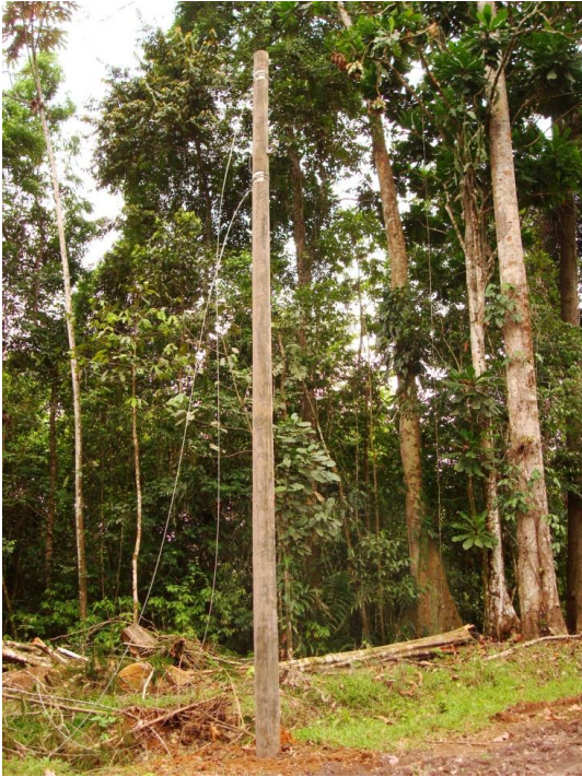
Photo of an electricity pole on the road to Crucitas
