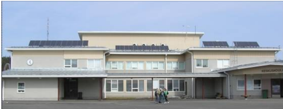
Figure 9: The PV system on the roof of the local school building in Saarijärvi [50].
