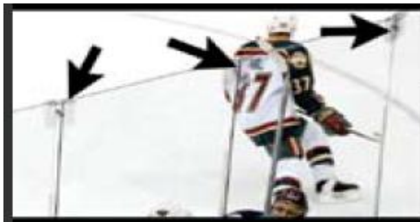
FIGURE 4. Clips allow each piece of protective glass to move independently upon impact (modified from Athletica 2011a).
