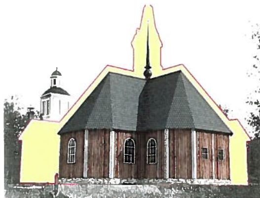
Figure 14. Overlay of the first phase. The yellow area presents the current size of the church.
