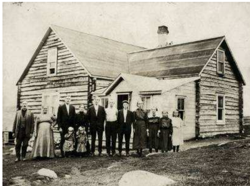
Illustration 5. The Alex Palo house in Wisconsin. This Finnish-American house in the turn of the 20 th century. It has a L-shaped plan, which was also common in Finland 1880-1910. Notice the shape of the porch roof – it was used for example in the surroundings of lake Päijänne in Finland. It is attached to the forms of Finnish vernacular tradition.
