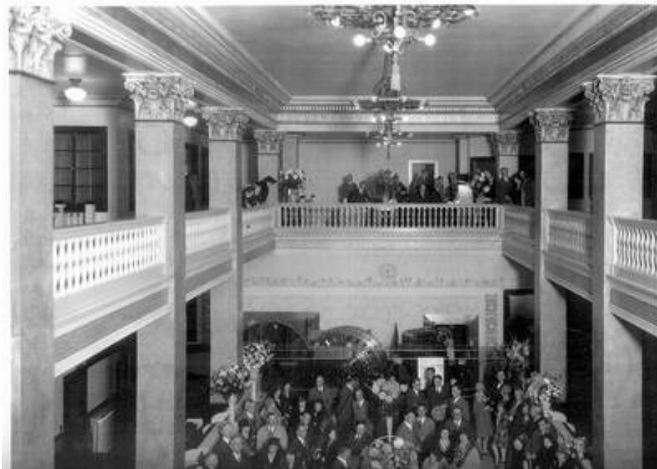
Illustration 37. The United States National Bank, designed John Wicks 1925. Constructed by Niemi and Company. Astoria, Oregon. Photos courtesy of Clatsop County Historical Society. Photo from: http://www.thebankerssuite.com/bankers_suite_history.html
