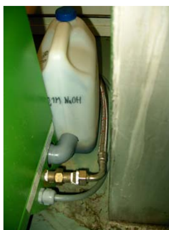
Figure 5. The condensation water was dropping directly into alkaline solution minimizing malodour formation into the room.
