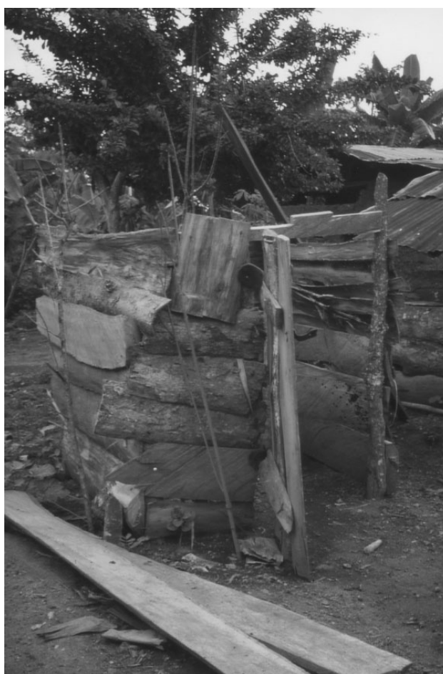
FIGURE 17 Bathroom hut in Oke-Ake
