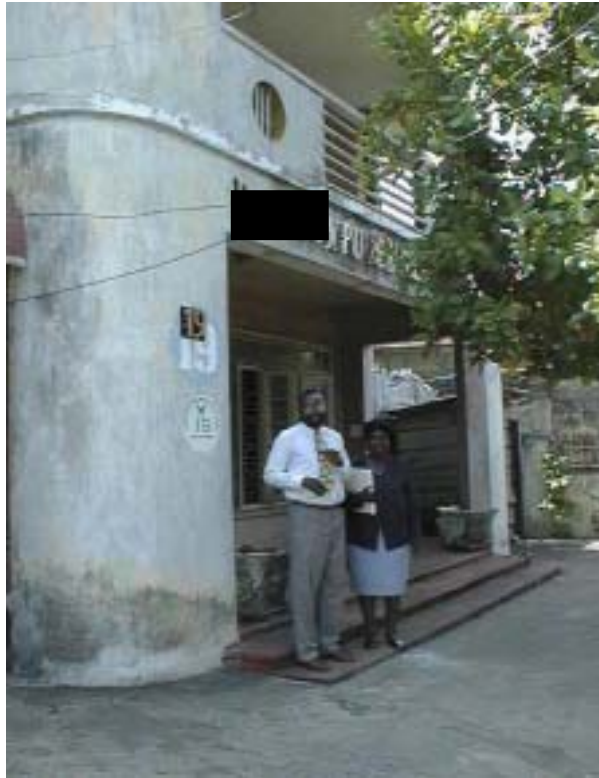
FIGURE 43 The company main building
