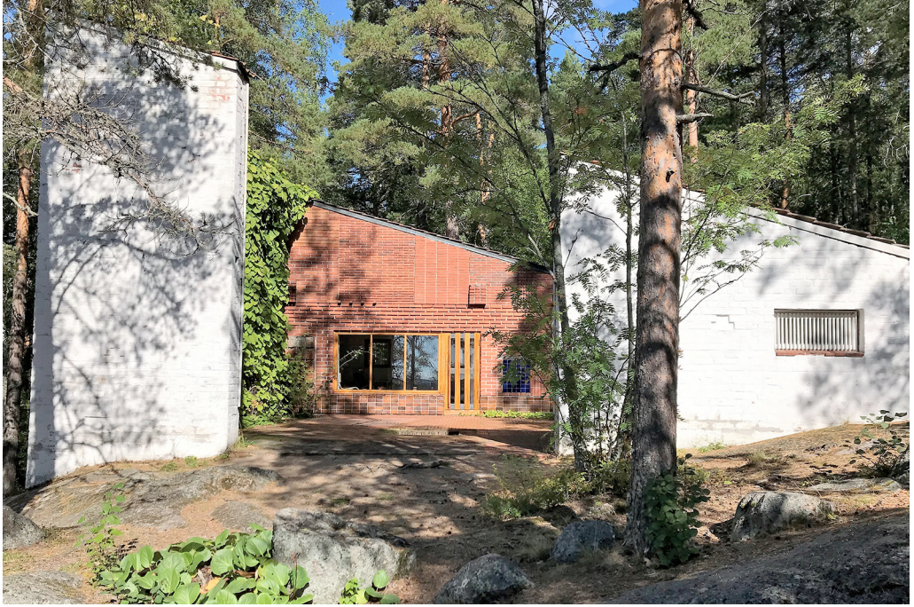
Fig. 1. The Experimental House was a summer house of architects Alvar and Elissa Aalto. The courtyard walls are covered with different brick and tile fields to test aesthetic and practical standpoints. Photo: author.
