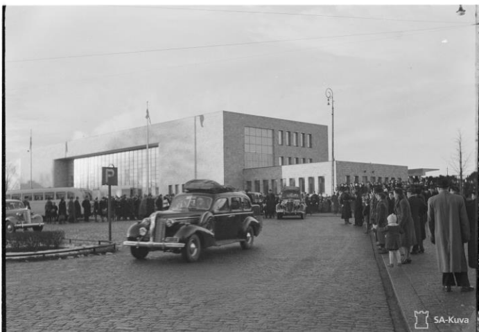
Photograph 1. Turku railway station.
