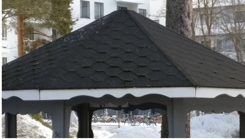
Figure 3: Lichen and moss growing on north-western (left) side, while south-western (right) side is almost clean.
