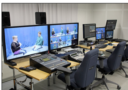
Figure 3: The control room
