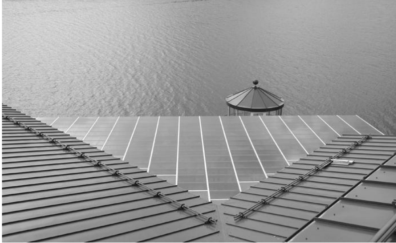
Figure 1: The terrace roof of the service station in Viitasaari [13].
