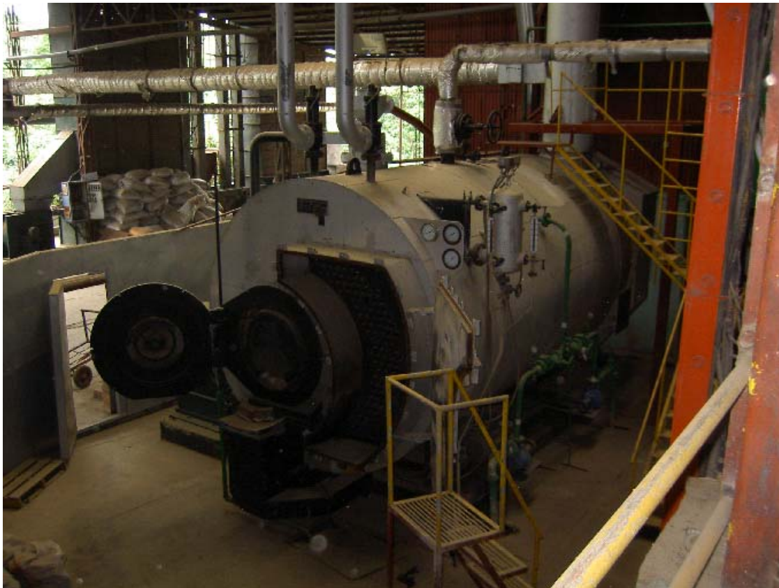
Figure 4. Boiler for biogas and coffee husks to generate heat for coffee drying.
