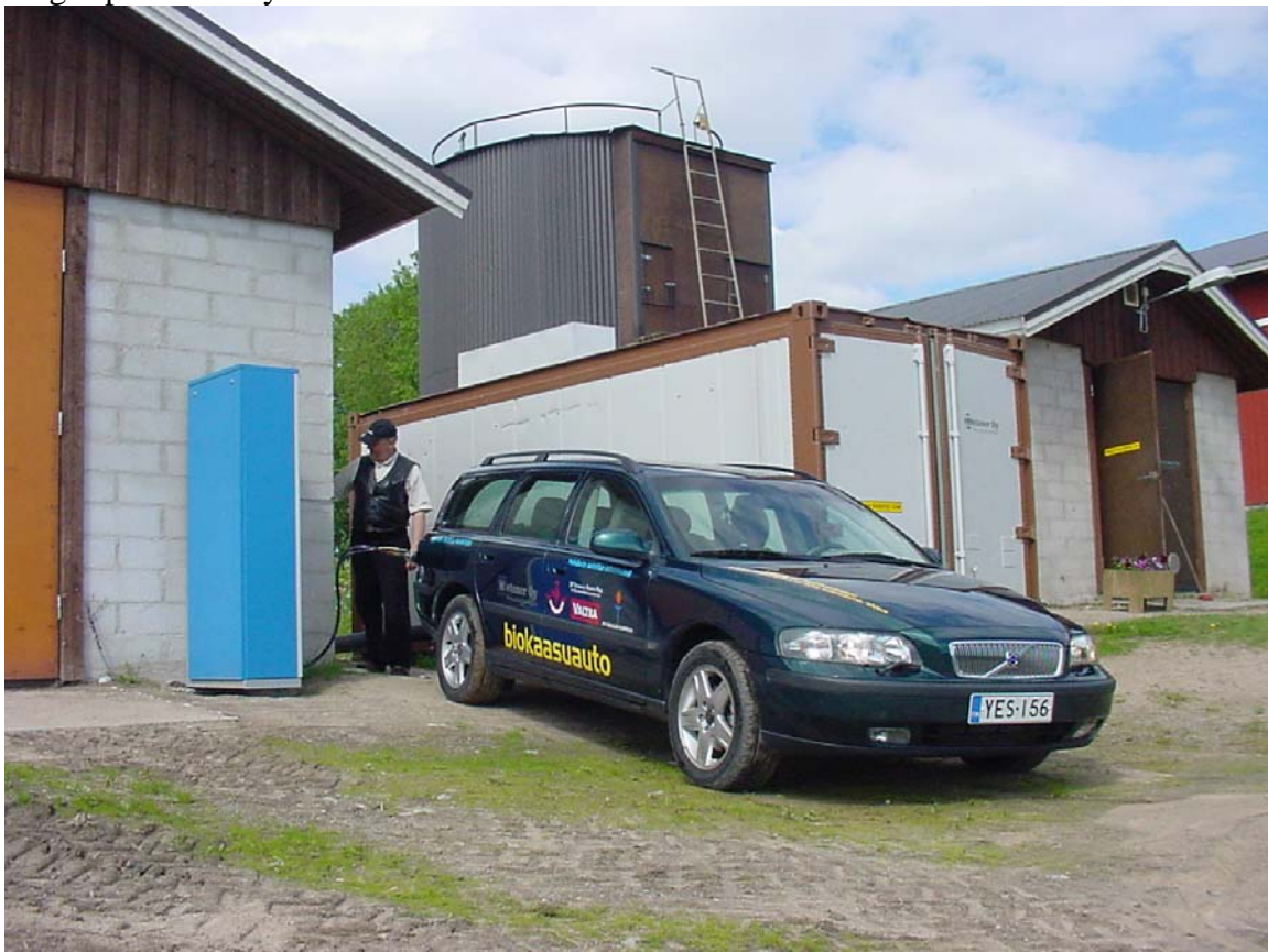
Figure 5.2. At Kalmari farm near Jyväskylä in Finland all electricity, heat and traffic fuel demands are met by self-produced biogas from cow dung and waste – and extra energy is sold for additional income. In this photo farmer Erkki Kalmari is fuelling his Volvo V70 Bi-fuel car by on-the-farm generated biogas methane. Biogas reactor is shown behind, as well as a building housing an Otto micro-CHP unit, and a container housing water scrubbing biogas upgrading unit for vehicle use. (Lampinen 2004)
