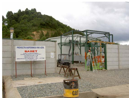
Figure 1. Electricity generation unit under construction in Río Azul in July 2004.
