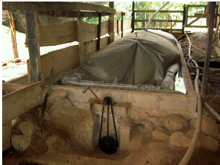
Figure 1. One of the bioreactors in the farm.
